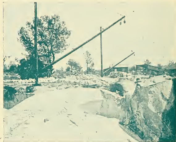
GRANITE QUARRY AT ROCKLIN.
